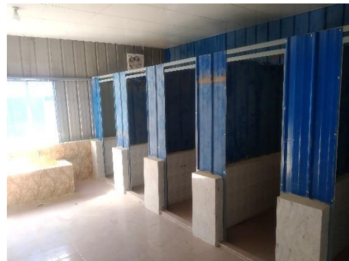
Renovation of NEPC Subcontractor labor shed
