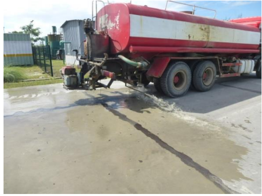
Water spraying at the project area
