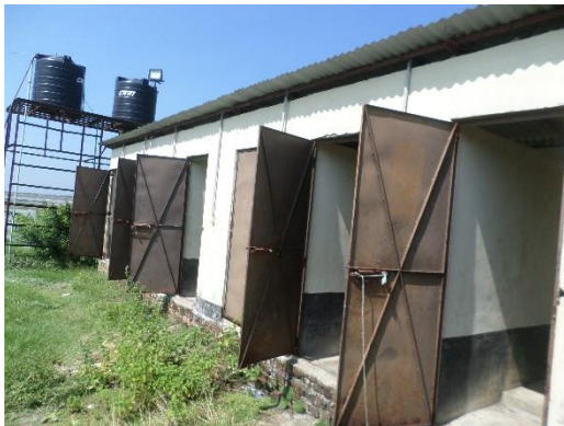
Toilets of NDE worker shed
