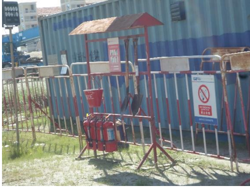
Fire safety kits available at project area
