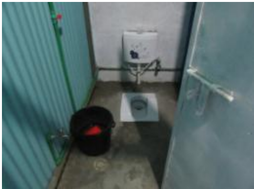
Toilet facility (NEPC)
