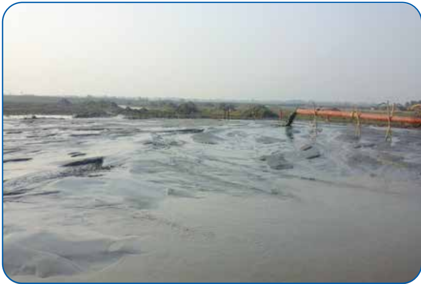
Land Development through Dredging for Payra 1320 MW TPP Project
