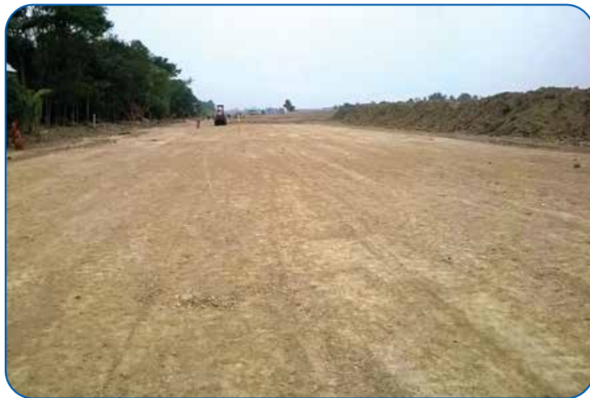
Embankment Work for Payra 1320 MW TPP Project
