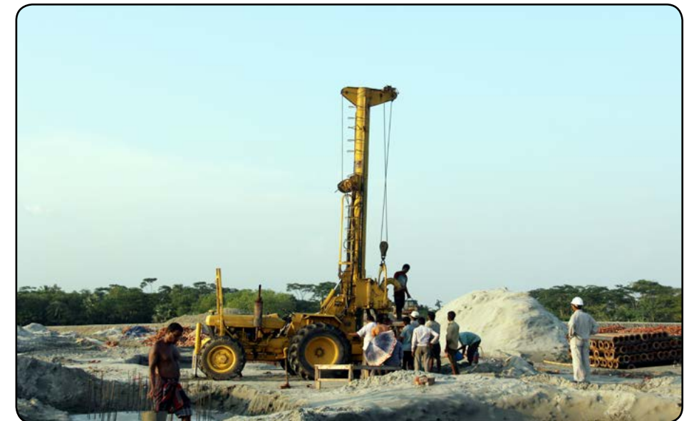
Water Well Drilling for Payra 1320 MW TPP Project
