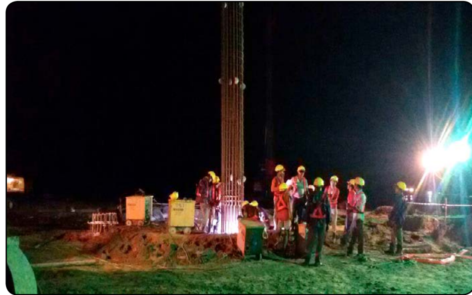
Installation of Rebars for Payra 1320 MW TPP Project
