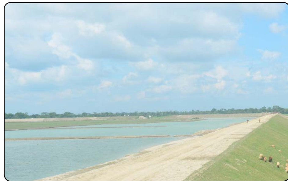
Embankment work for Payra 1320 MW TPP Project
