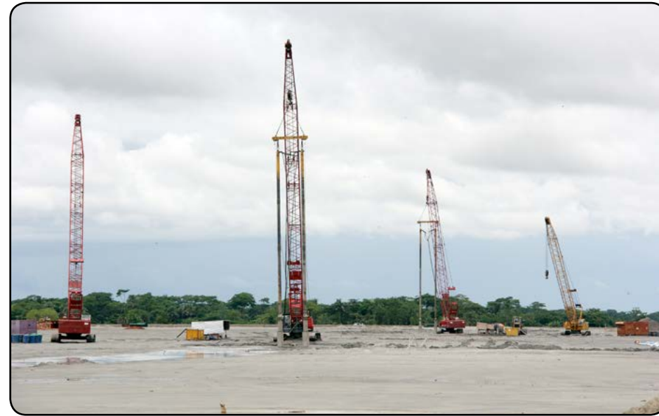
Soil Improvement Work for Payra 1320 MW TPP Project
