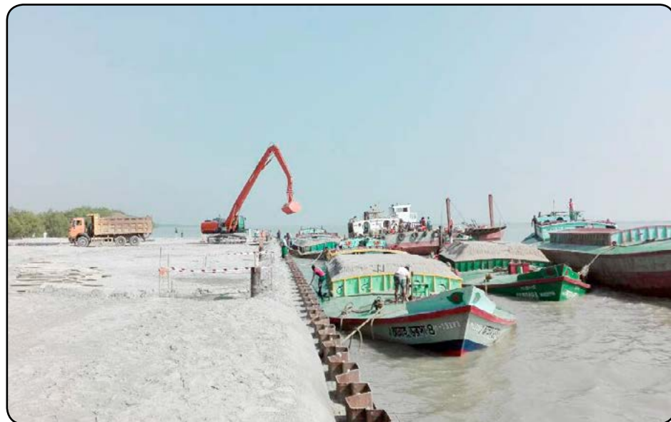
Temporary Jetty for EPC Work for Payra 1320 MW TPP Project
