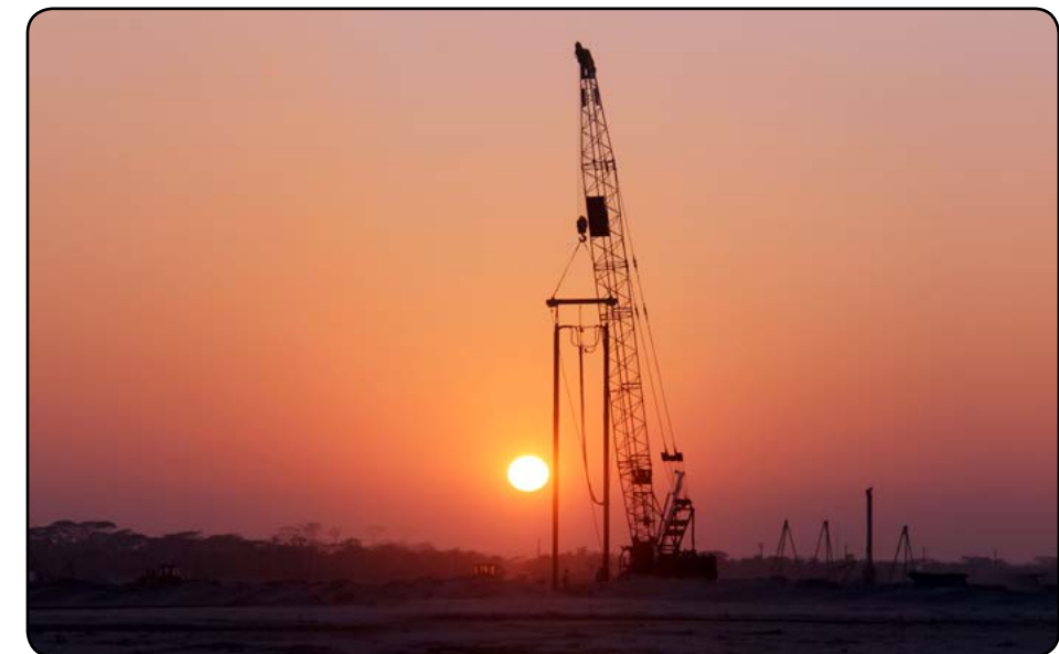
Soil Treatment for Payra 1320 MW TPP Project
