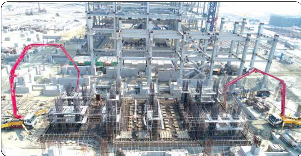
Concrete Casting of TG Pedestal for Payra 1320 MW Thermal Power Plant
