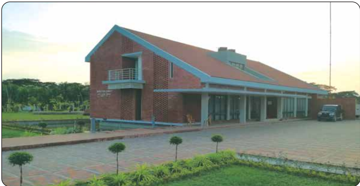
Inspection Bungalow for Payra 1320 MW Thermal Power Plant Project
