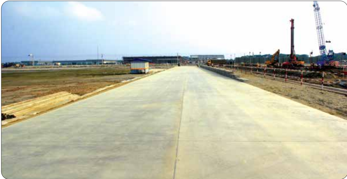
Internal Road at the Payra 1320 MW Thermal Power Plant Project Site
