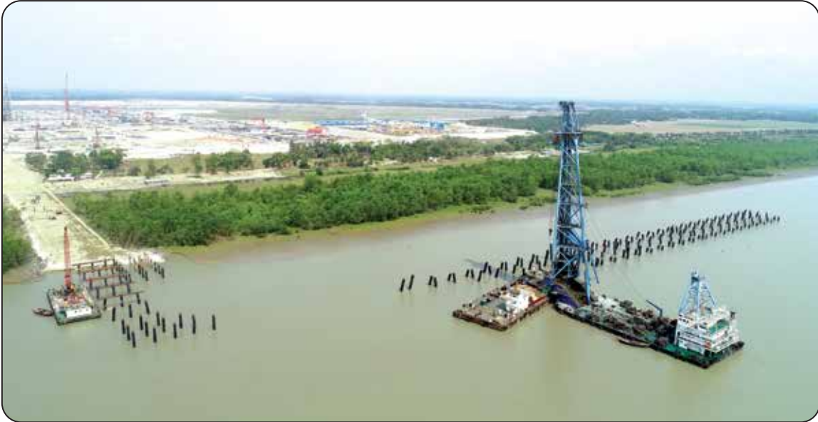
Steel Piling in Coal Jetty for Payra 1320 MW Thermal Power Plant
