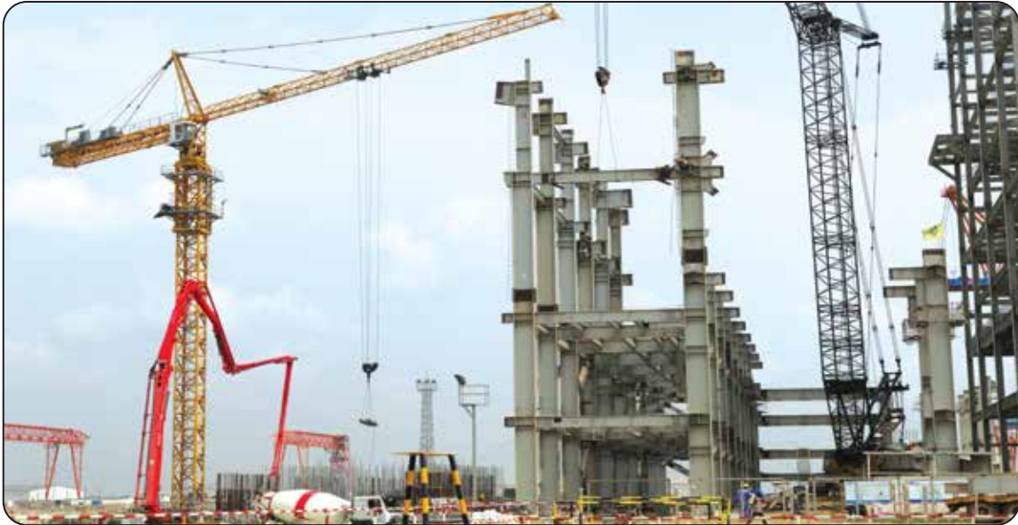
MPB Steel Structure for Payra 1320 MW Thermal Power Plant
