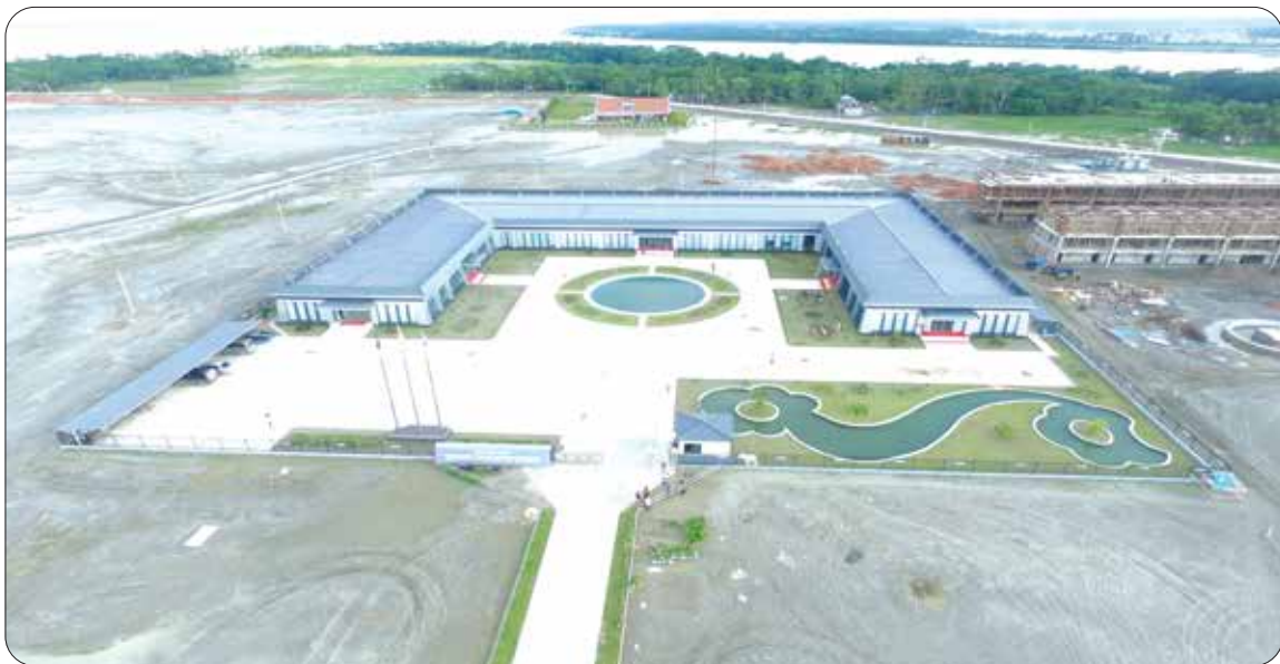
EPC Office for Payra 1320 MW Thermal Power Plant Project
