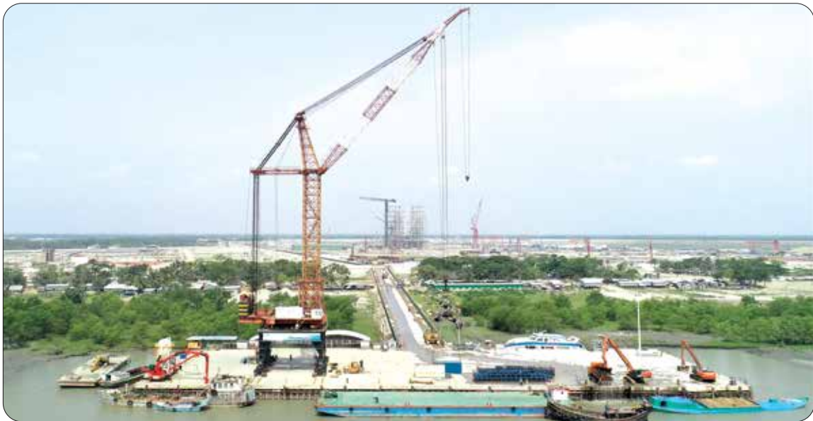
Service Jetty for Payra 1320 MW Thermal Power Plant
