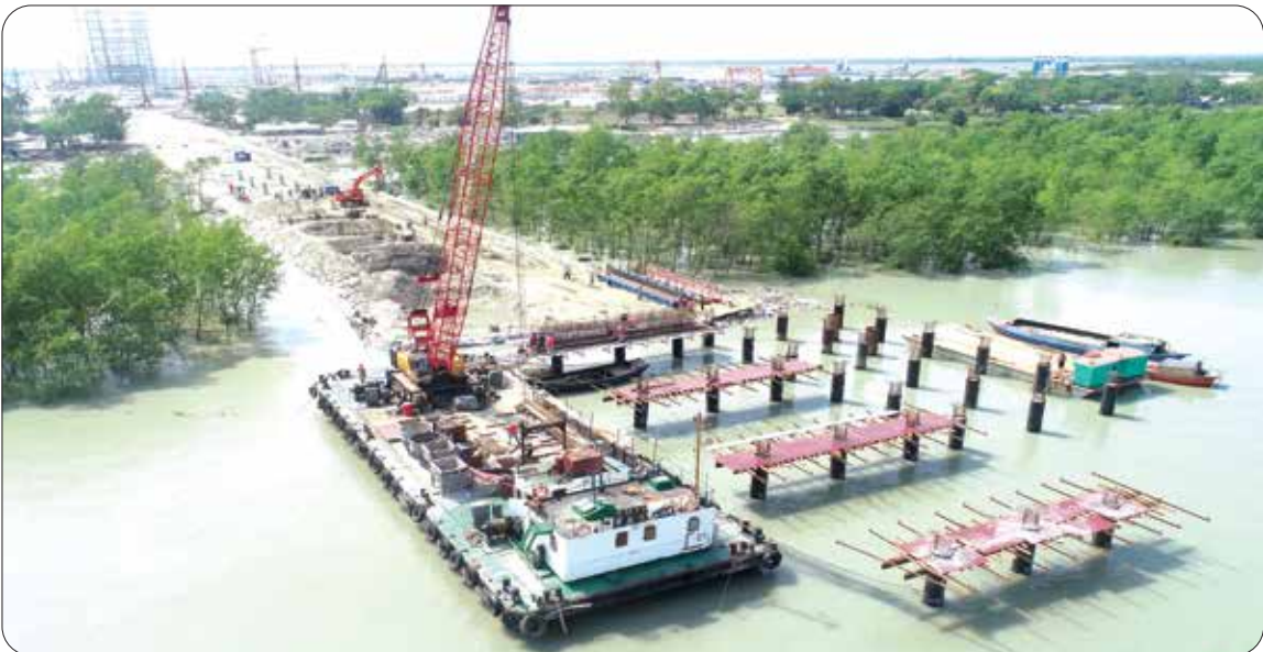
Construction of Coal Jetty for Payra 1320 MW Thermal Power Plant
