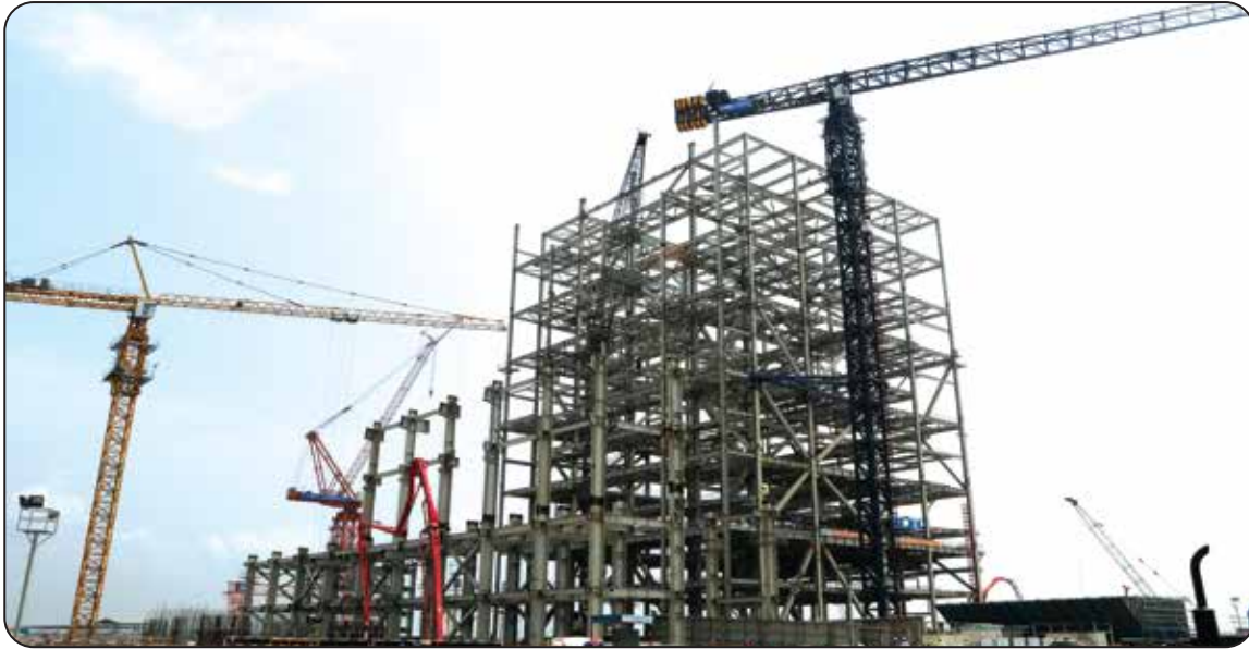
Boiler #01 Steel Structure Erection for Payra 1320 MW Thermal Power Plant
