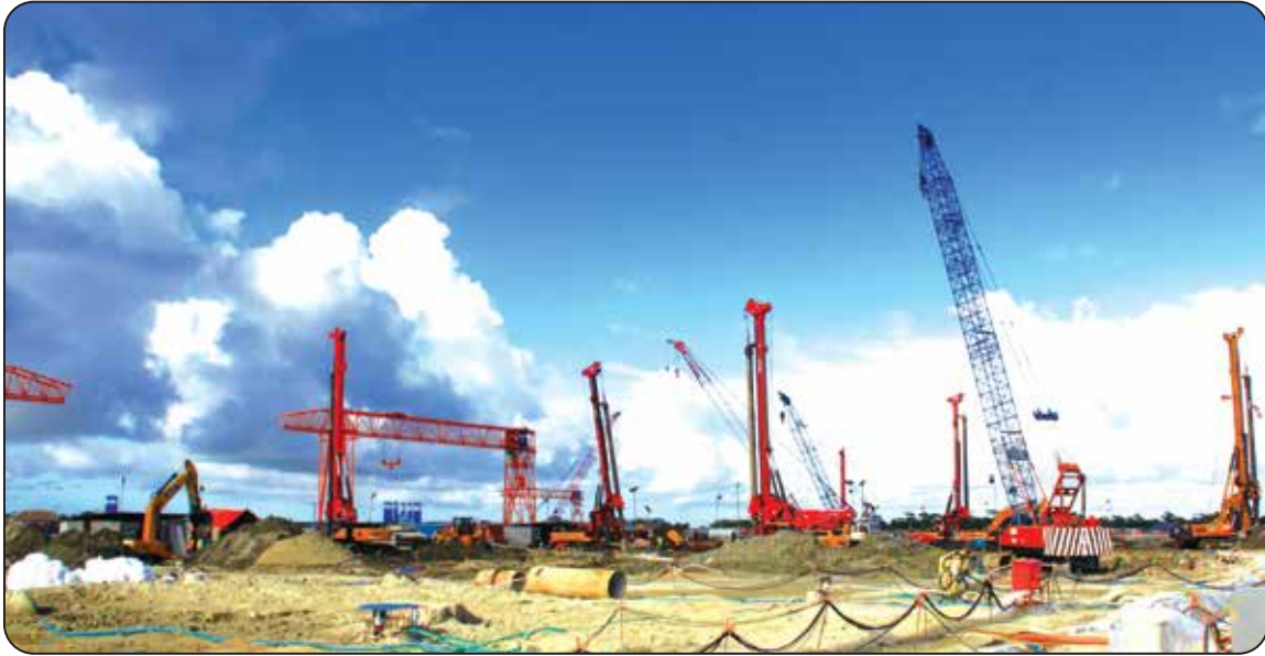
Service Pile Work for Payra 1320 MW Thermal Power Plant
